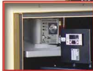
SMART FPS-DX In Generator Enclosure
